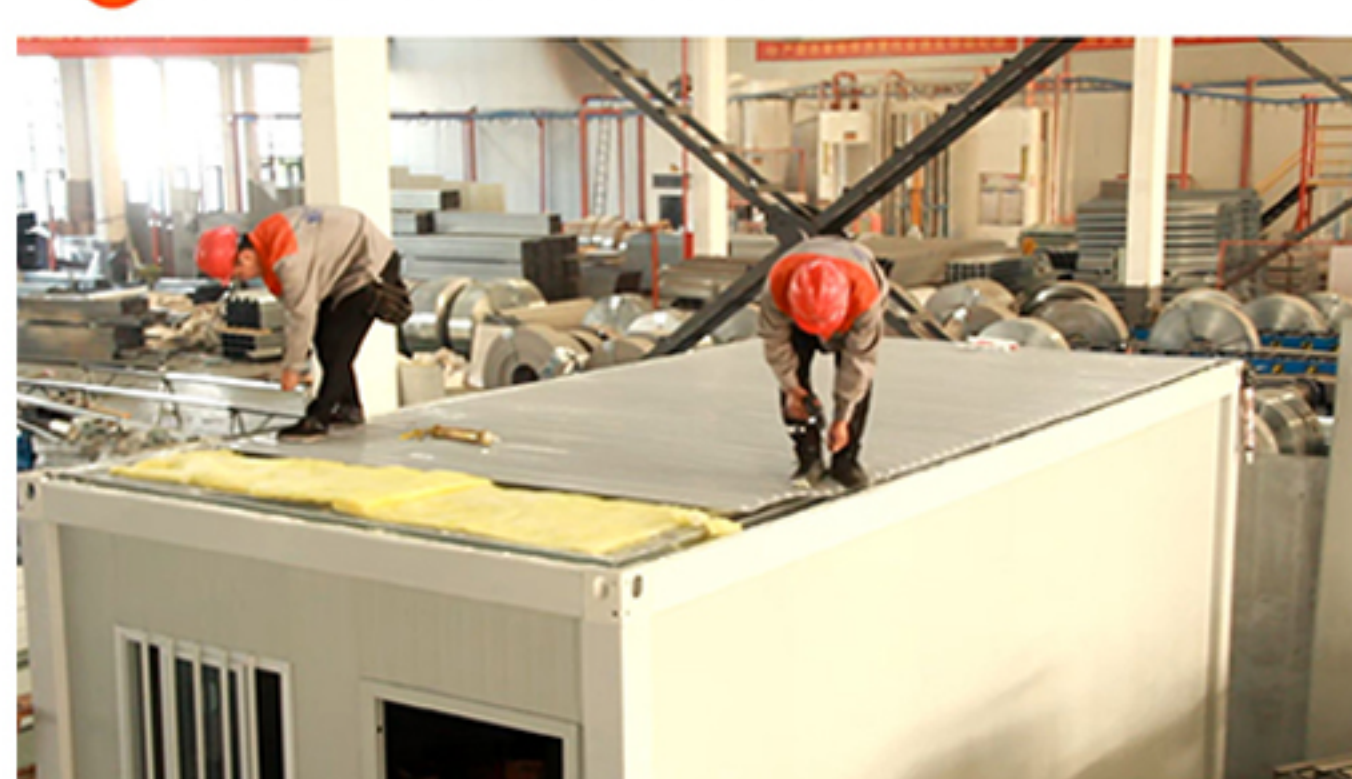
10 Install roof tiles and put sealant on screws
