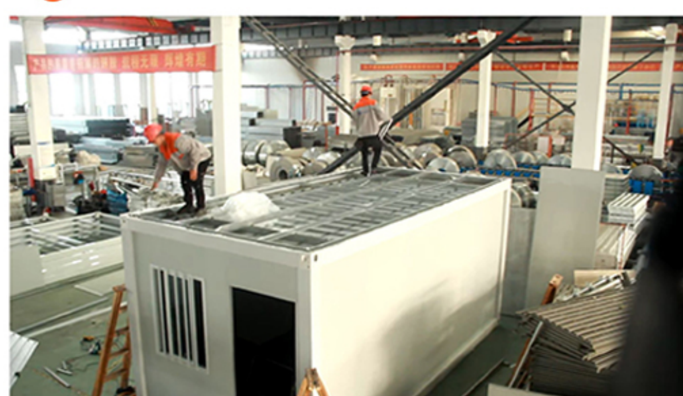
8 Install ceiling tiles and roof purlins
