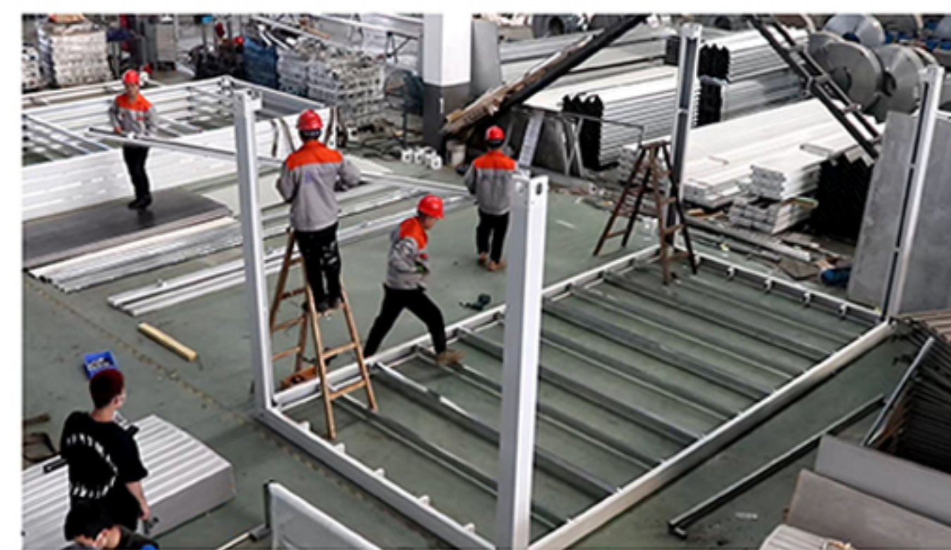
3 Install columns, make sure it's vertical
