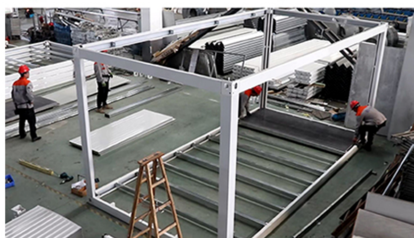
4 Put floor board on floor purlins
