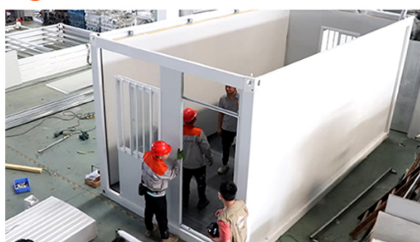
7 Install doors and windows
