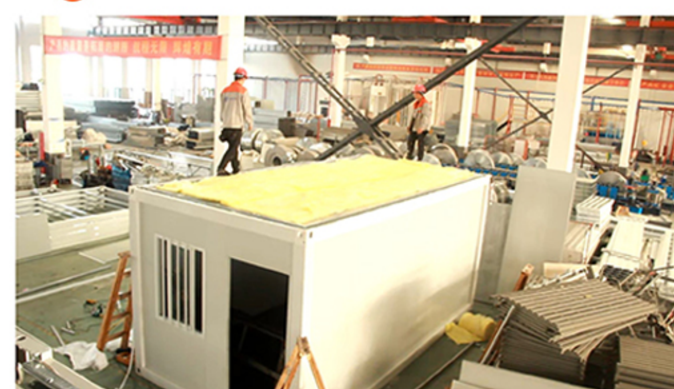
9 Put insulation layer on the roof purlins
